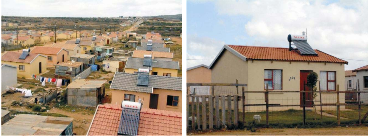
Figure 3: Low pressure SWH installed on Government housing (Zanemvula SWH pilot project)
